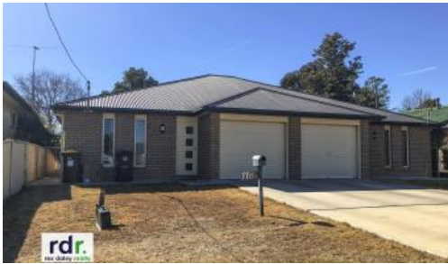
118A & 118B Mansfield St, Inverell
